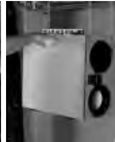
figure 5.4 When completing the procedure make sure that the HRV or ERV is leveled.
