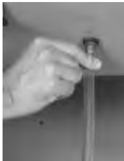
figure 8.2 Insert condensate line.
