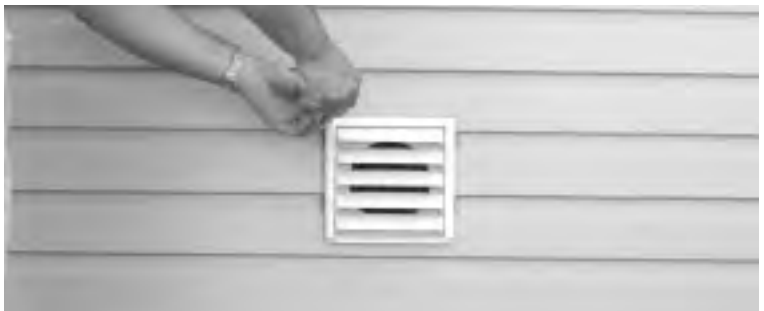
figure 10.4 Install outside hoods.
