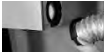
figure 6.1 Mount flex to HRV/ERV.
