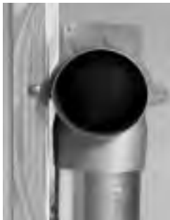
figure 11.2 Stack head elbow.
