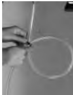
figure 8.3 Make a loop in condensate line.
