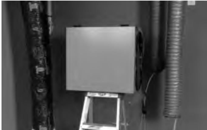
figure 5.1 Place HRV/ERV on a stepladder.
