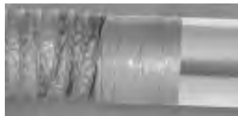
figure 6.2 Mount flex to rigid duct.
