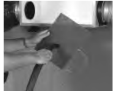
figure 17.2 Vacuum the Filters
