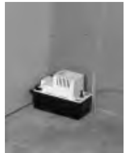
figure 8.4 Use a condensate pump if you don't have access to the floor drain.
