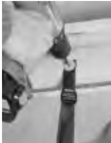
figure 5.2 Attach your four straps to the floor joist making sure that you attach thru the washers and the grommets.
