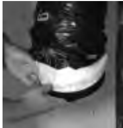
figure 7.3 Insert insulation inside the collar.
